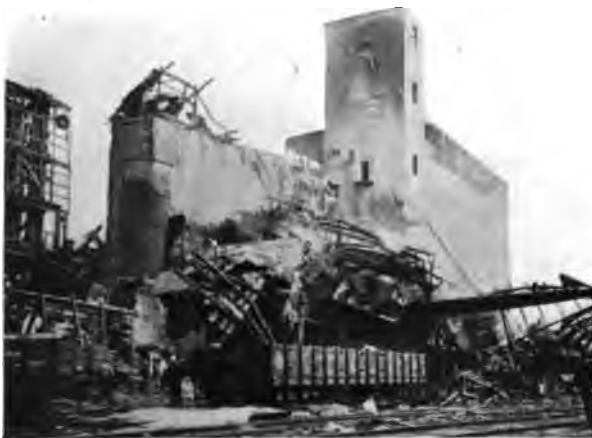
Fig. 3. Result of Dust Explosion in Feed Mill and Grain Elevator.
